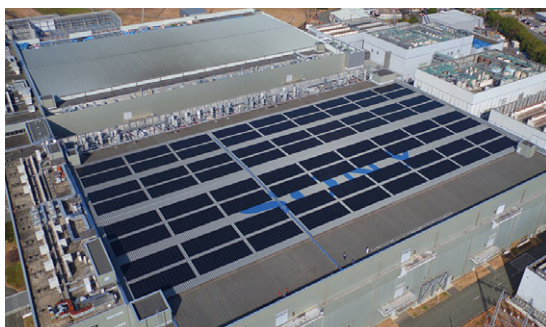
Solar power generation equipment (Kumamoto Technology Center, Sony Semiconductor Manufacturing), which began operation in 2019
